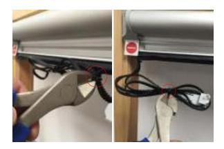
6. Using a pair of side cutters or similar, cut the tie holding the two loops of belt together, then cut the tie to release the loops of belt.
