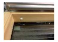
1. Remove the white plastic plug from top left corner of sash.
