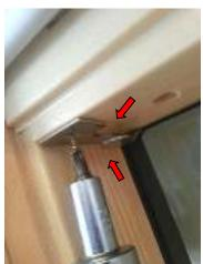
2. Screw the left-hand mounting bracket into place in the top corner of the sash, making sure the front edge is level with the edge of the sash timber and the side is flush with sash side.
