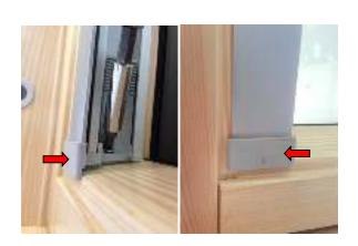
12. When siderail is in position, fix it in place with one of the screws provided. Make sure siderail is pushed up tight against the front edge of the sash and tight against the side of the sash.
