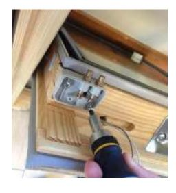
13. Unscrew the two 15mm screws from the Blind Contact.
