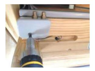
17. Replace the lid back onto the Blind Contact and secure into place with screw.
