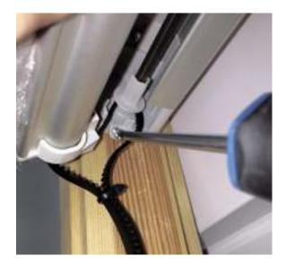
8. Pull down the blind fabric from the cassette slightly to expose the fixing screw ports. Using two of the screws provided, secure the blind cassette to the sash as shown, one screw on each side.
