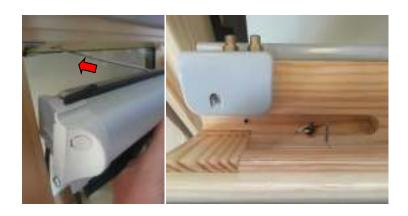
4. Open the window using the vent flap handle and feed the wires from the top of the blind cassette through the 8mm hole in the sash. Pull as much of the wire through the hole as possible, and before closing the window again, please ensure the wires are tucked away securely in the recess provided.
