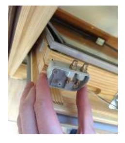
14. Remove the Blind Contact from the sash.
