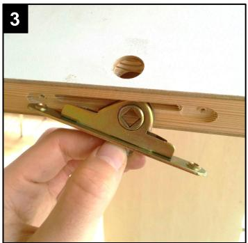
Remove the lock mechanism from the end of the door.
