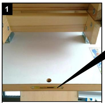
Expose the lock mechanism by opening the loft ladder door. The lock is located in the end of the door, below the steps.
