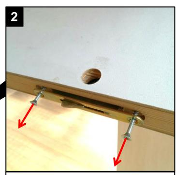
Remove the two screws at either end of the lock which secure it to the door.
